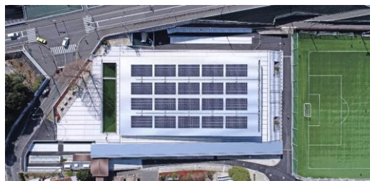
Solar Panel on roof of swimming pool building on campus
