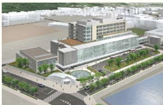
The New Building opened on 4 January 2011 contains the Organ Center incorporating almost all outpatient departments, as well as in-patient facilities for the Perinatal and Mother/Child Medical Center, the Pediatric Medical Center, the Heart Center and the Digestive Tract Center, and is directly connected to the Fukudai-mae station of the Nanakuma subway line. Adjacent to it is the Medical Hall, with seating for three hundred, while the Medical Fitness room is situated on the basement level, providing an integrated approach to health, nutrition, pharmaceutical creation and medicine.
